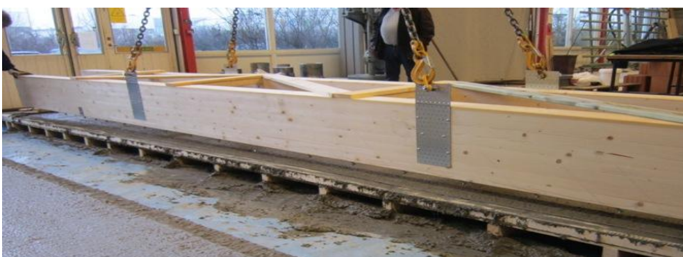
Fig. 10. Insertion of the glulam beams in the fresh concrete
