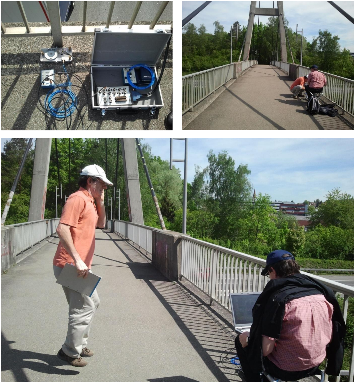
Figure 1. Dynamic test in a concrete bridge
