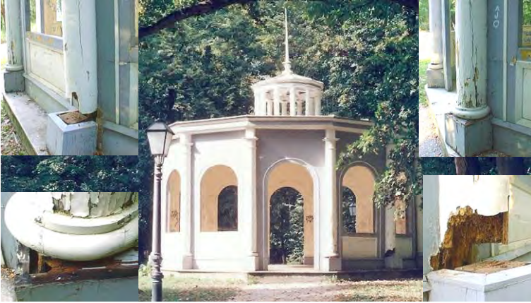
Fig. 2 State of the Pavilion «Echo» before reconstruction
