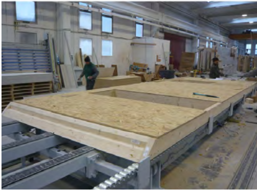
Fig. 1: Timber frame wall assembling
