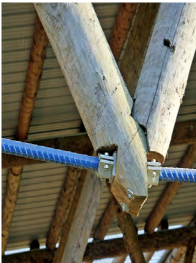
Fig. 1 Round wood truss joint
