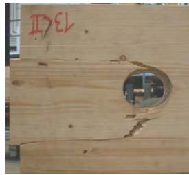
Fig. 5 Combined shear and tensile failure in prestressed
