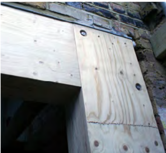
Fig. 1 LVL Portal Frame Connection (Courtesy of Webb Yates Engineers)
