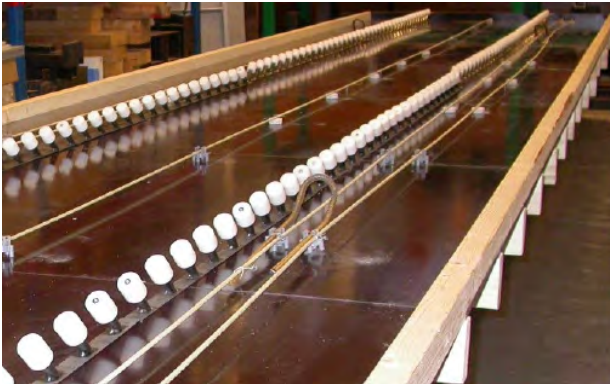
Fig. 3: Shear connectors in T12 specimens (note the white plastic plugs inserted on the top of the tubes to prevent concrete from entering in the tubes during casting)
