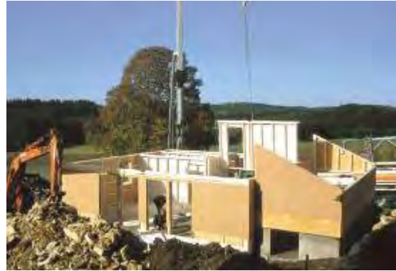
Fig. 2 :Timber frame walls positioning on site
