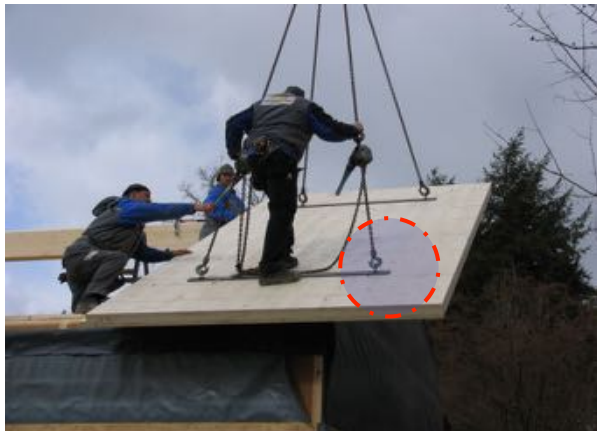
assembling of roof elements
