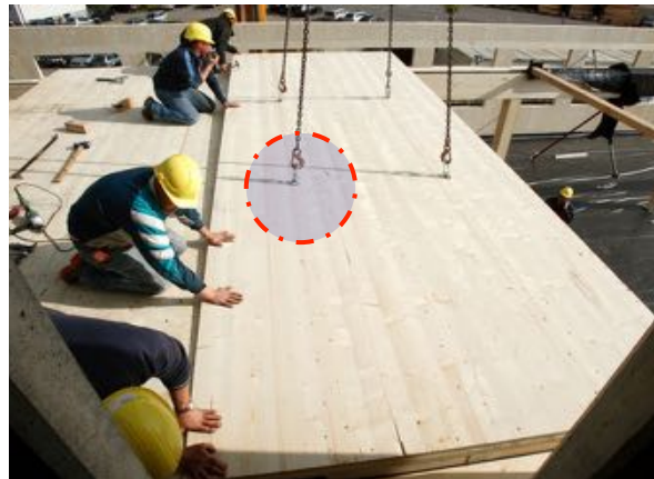
assembling of ceiling elements
