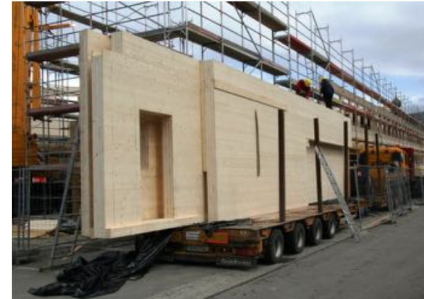
discharging (building site)
