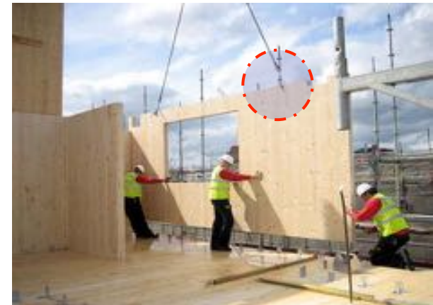
assembling of wall elements
