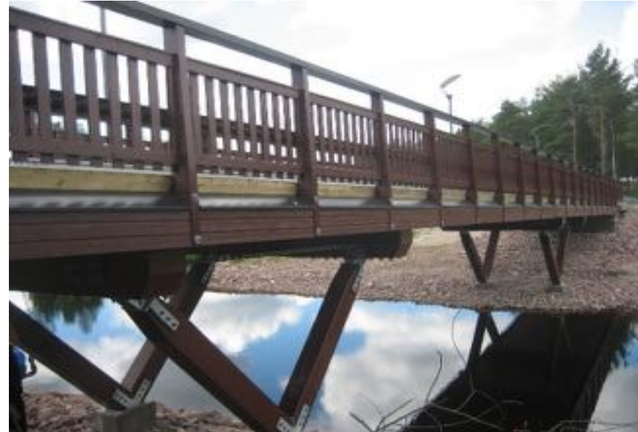
Railing with both balusters and top rail made of wood
