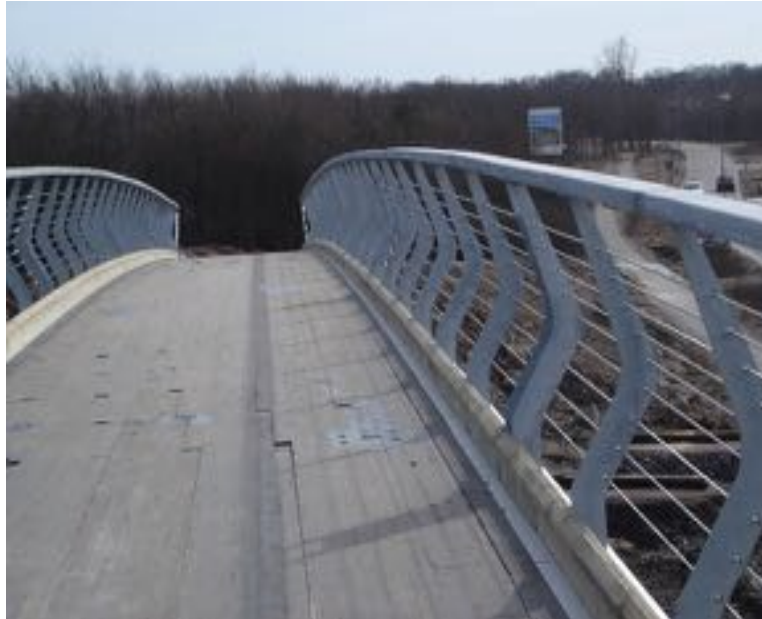
Railing with balusters of steel and a top rail of wood
