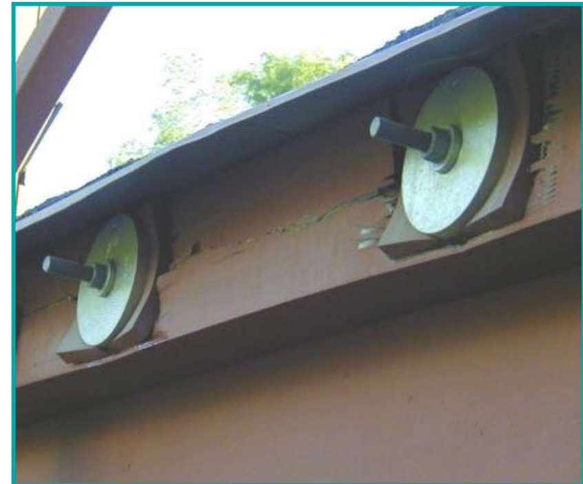
Lusbäckenbron, Borlänge – Stress-laminated box-beam Bridge
