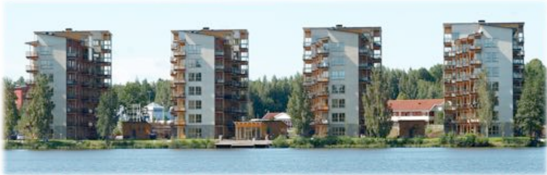
Limnologen 7-storey, Sweden
