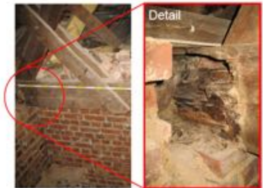
Figure 19: Heart rot damaged head in load-bearing joist at opened brick work
