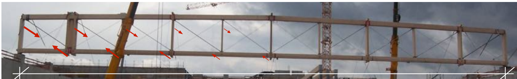
Span L = 78 m, Load F = 1100 tons (60 trucks)
