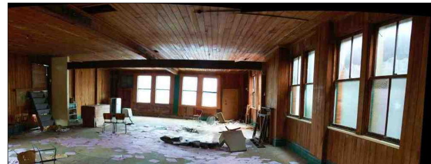
First floor interior
