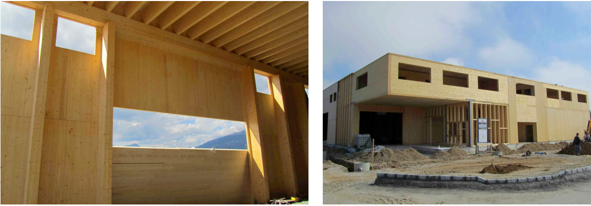
Fig 1: Ekoprodukt storage hall. Bracing system (left), cantilever (under construction) on the right.
