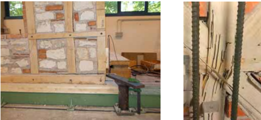
Fig. 2: Rocking mechanism on Baraccato sample and joint collapse in the Gaiola wall.
