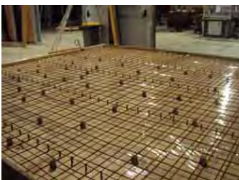
Fig. 2: TCC floor assembling.
