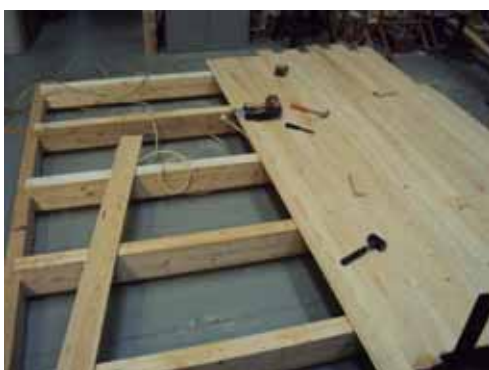
Fig. 1 Timber floor assembling.
