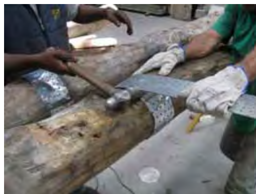
Fig. 3: Application of steel strips
