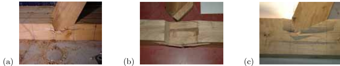
Fig. 2: Experimental failure patterns observed:
