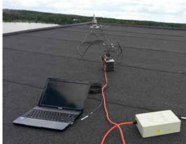
Fig. 2: The test system measuring a single point, from top: accelerometers, data acquisition system, laptop and power supply
