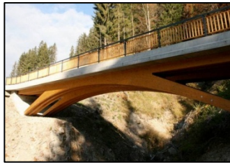
Ragoztobel Bridge, Switzerland
