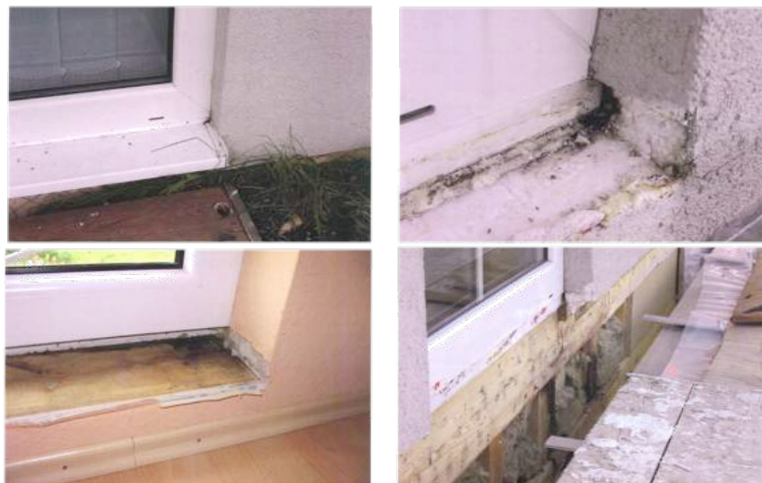
Fig. 33 Example of bad moisture-proofing design: a small leakage at the corner of an exterior windowsill led to expensive moisture damage of the exterior wall and parts of the wooden slab
