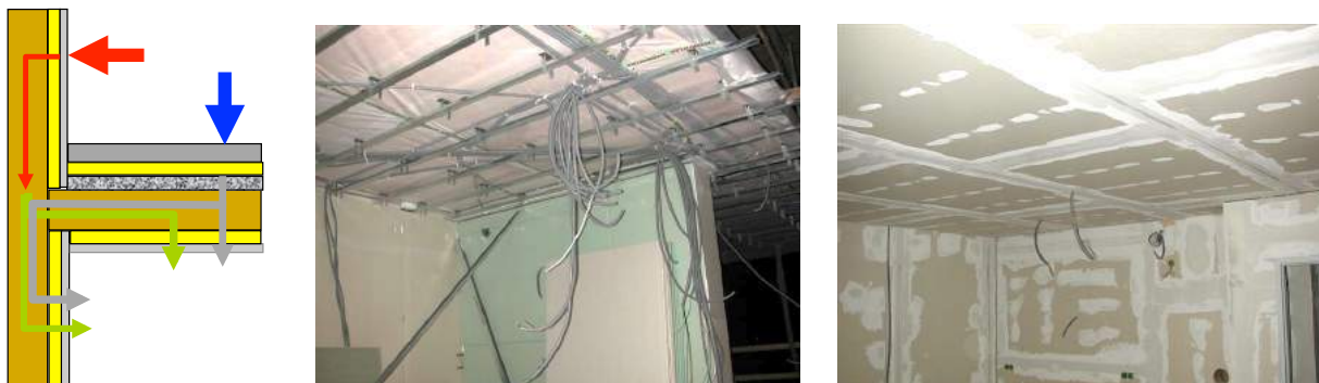
Fig. 82 “Room-in-room” construction system
