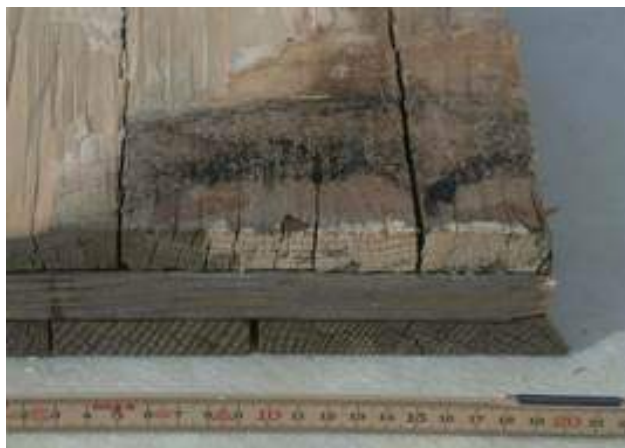
Fig. 3 CLT can be damaged or destroyed by extended action of humidity.
