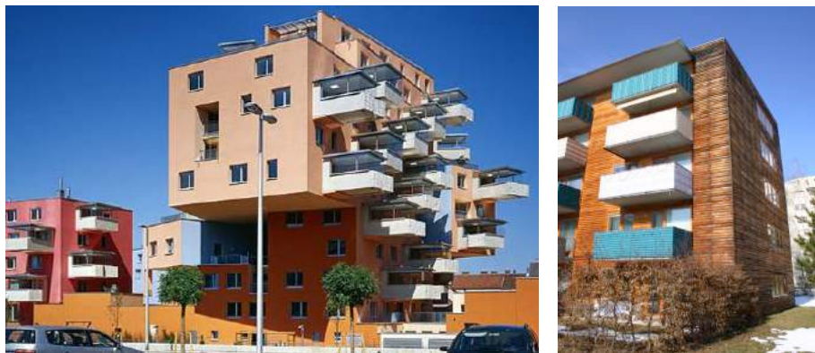
Fig. 29 left: Extremely weather exposed façade; right: Wooden façade with and without cantilever roof
