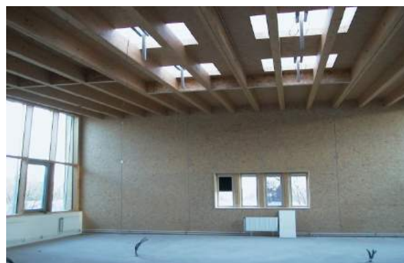
Fig. 24 Special solutions for the centre of Building Technology at Graz University of Technology: Trussed CLT system as roof construction for the great testing hall (left) GLT-CLT ribbed plate as roof construction for the offices (right)
