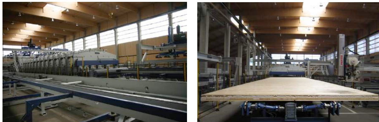
Fig. 7 Hydraulic surface and edge pressing device (left); unloading of ready produced CLT (right) (© Minda-Industrieanlagen GmbH / DE)
