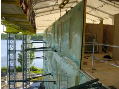
Fig. 26 Weather protection Limnologen, Växjö. Source: SP Technical Research Institute of Sweden, Per-Eric-Eriksson
