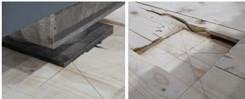
Fig. 9 Intense indentations in the area of the load application
