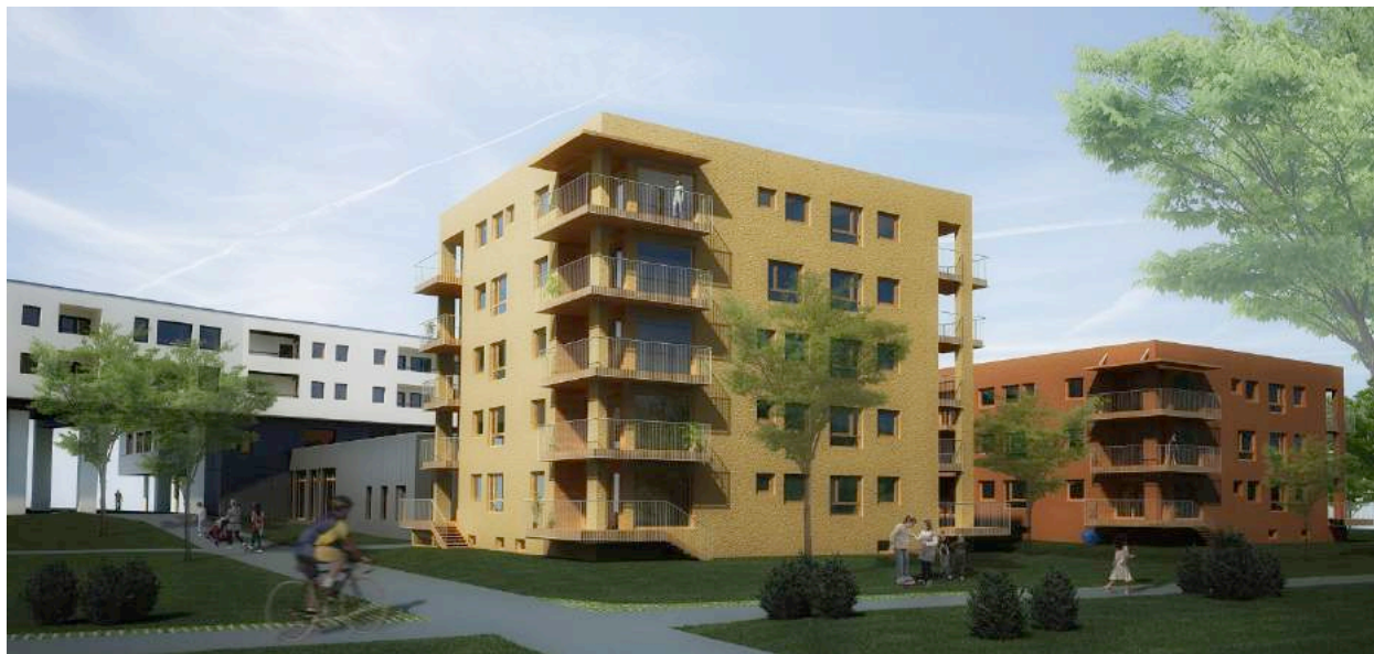
Fig. 25 Image of a five storey residential building of the project “Peter Roseggerstraße“ [22]
