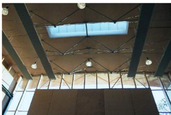
Fig. 24 Special solutions for the centre of Building Technology at Graz University of Technology: Trussed CLT system as roof construction for the great testing hall (left) GLT-CLT ribbed plate as roof construction for the offices (right)
