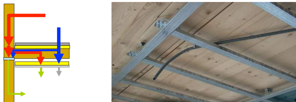
Fig. 80 Elastic membrane bearing below slab supporting surface- suspended ceiling with resilient bars
