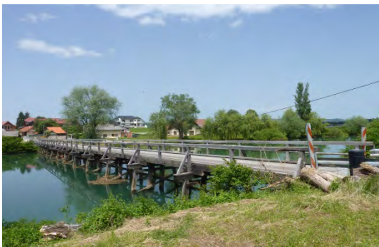
Figure 1: Timber bridge over Krka river
