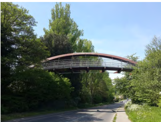
Figure 2 Black Dog Bridge from the road
