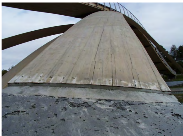
Figure 11: Arch of Leonardo Bridge before the cladding (NPRA)
