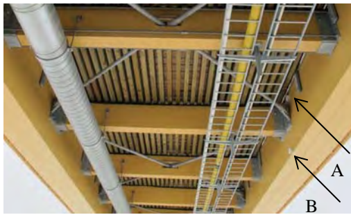
Figure 2: Bridge from underside with sensors
