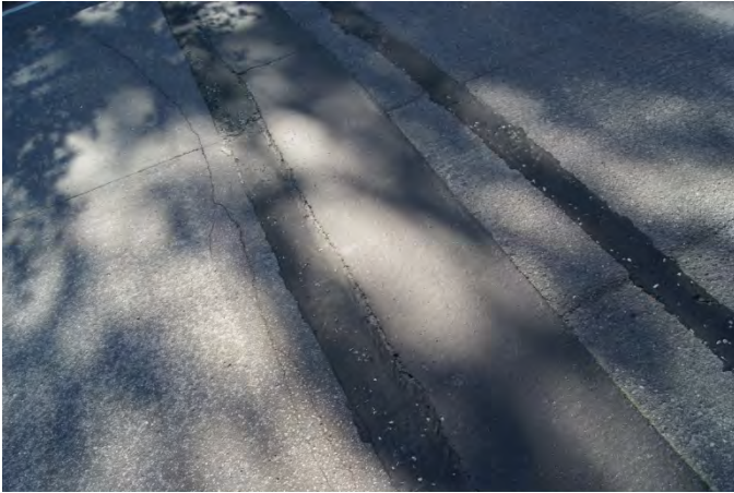
Figure 15: Støpeasfalt (left side) used on Møllendammen bridge
