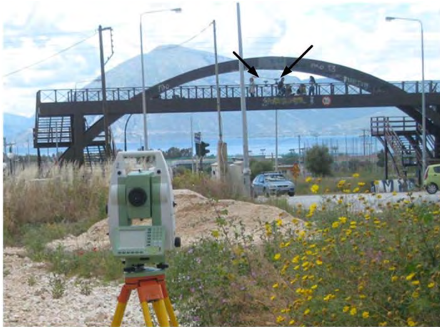
Figure 1: Side view of the Kanellopoulos pedestrian timber bridge in Patras. A Robotic Total Station (RTS) is shown in the foreground, while arrows indicate collocated sensors, including RTS reflectors and accelerometers.
