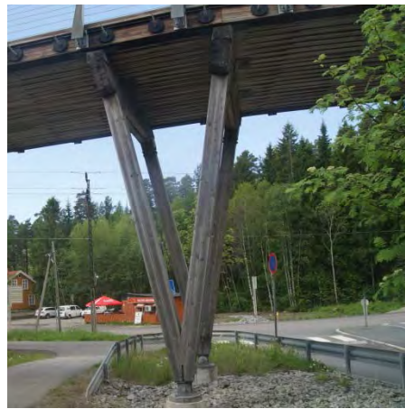
Figure 9: V-shaped column (Sørliveien bru)
