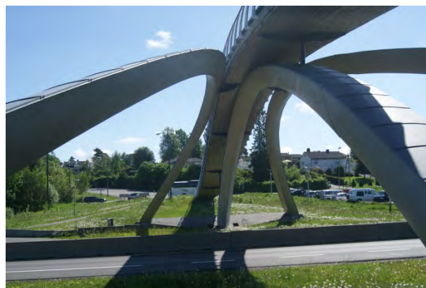
Figure 12: Arches of Leonardo Bridge after the zinc cladding
