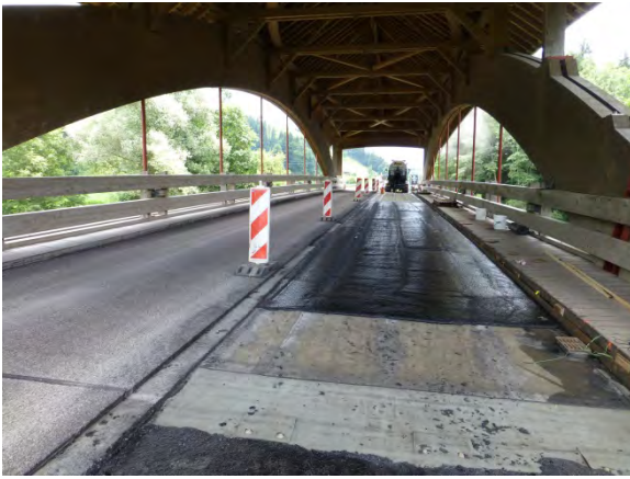
Figure 25: Picture of the Bubenei Bridge during the asphalt coating
