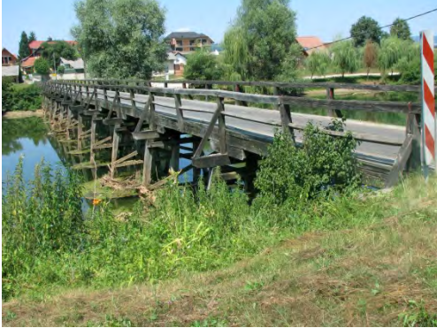
Figure 14: timber bridge over Krka river in Loke
