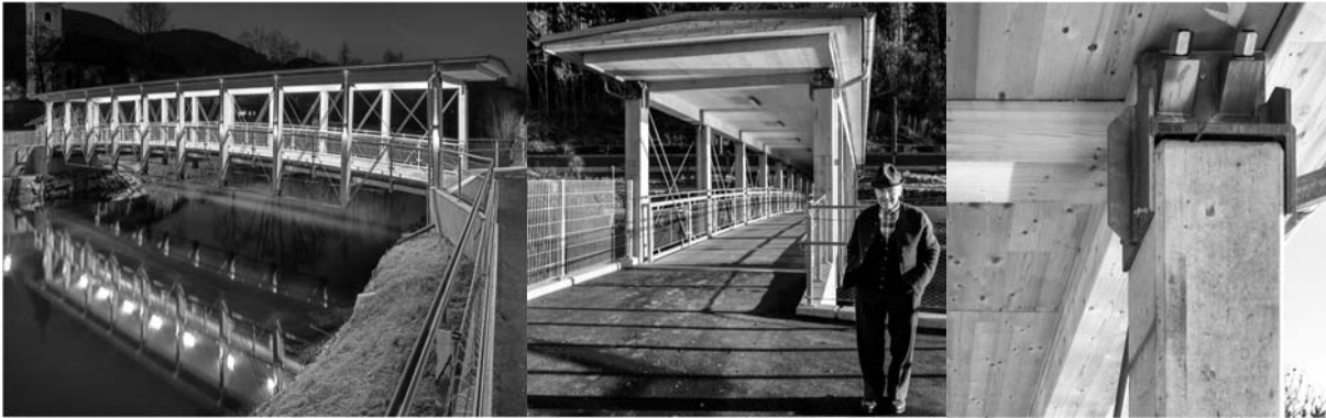
Figure 9: Impressions of the timber footbridge ‘Truss Bridge Kindberg’
