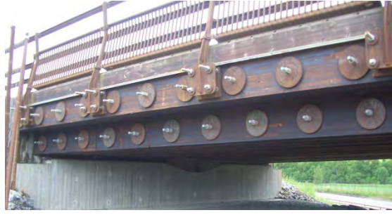
Figure 3: Bridge with two rows of pre-stressed rods
