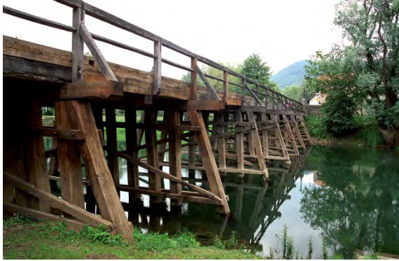
Figure 4: Kostanjevica na Krki: north bridge
