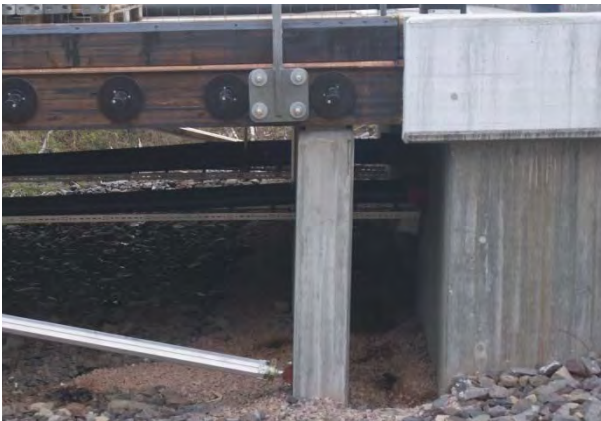
Figure 8: Free space below intersection between timber and concrete (Åsta bridge)
