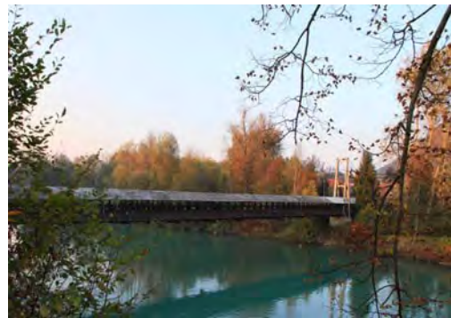
Figure 2: Timber bridge over Sava river in Vikrče
