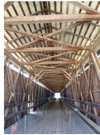
Figure 5 Walkway of Knight Ferry Covered Bridge
