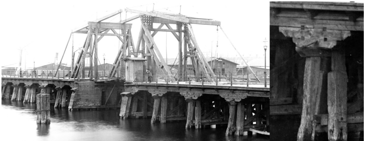
Figure 6: Third of the presented timber bridges of Szczecin is Most Dworcowy built in 1850-1852. This bridge existed as a timber bridge up to 1898. Photo 1890, [15]
