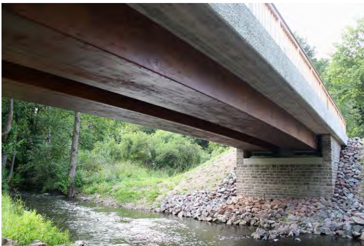
Figure 1: TCC Bridge „Birkbergbrücke“ Germany
