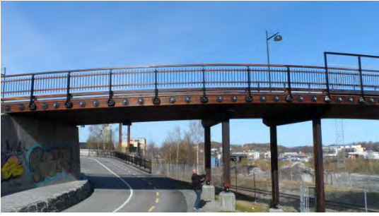
Figure 2: Bridge with one row of pre-stressed rods
