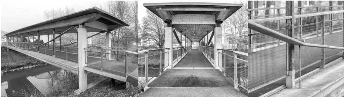
Figure 7: Impressions of the timber footbridge 'Raabsteg Feldbach'
