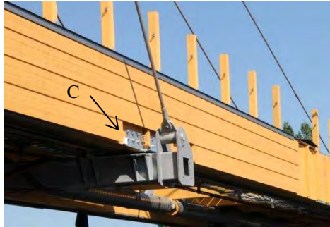
Figure 4: Moisture sensor on beam outside, bottom (C)
