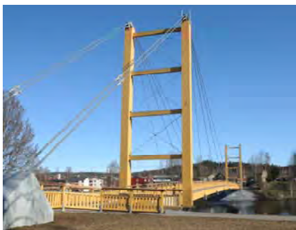
Figure 1: The Älvsbacka Bridge
