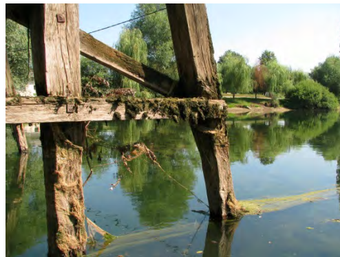
Figure 17: Reduced cross section of pillars
