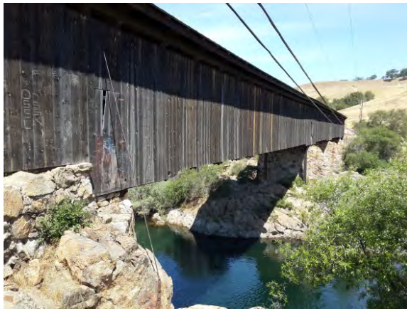
Figure 4 Knight Ferry Covered Bridge from outside
