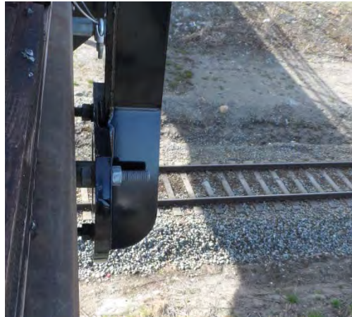
Figure 7: Good detail with respect to standing water
