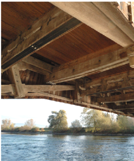
Figure 1: Wooden bridge, Sins, bottom view
