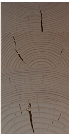
Figure 1: Shrinkage cracks in glulam
