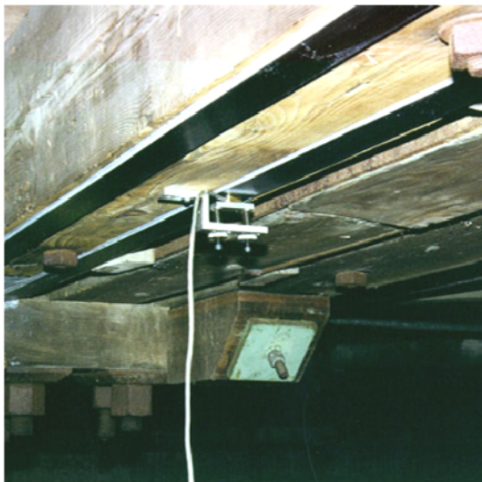
Figure 3: Externally applied plates
