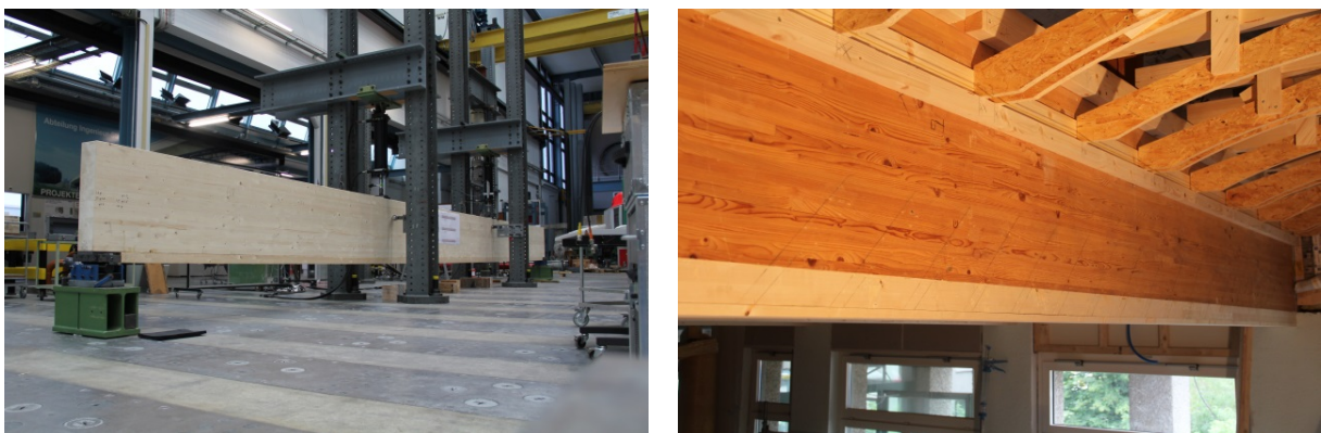
Figure 4: Application of (reinforced) additional lamellae for the strengthening of beams. Right hand side: laboratory tests, left hand side: application in practice.
