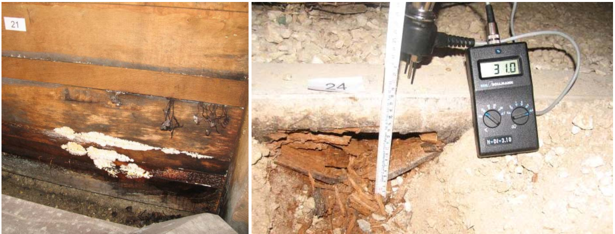
Figure 4: Fungi attack due to a high moisture content Figure 5: Degradation depends on high moisture content
