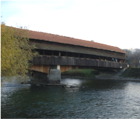
Figure 5: Wooden bridge, Sins
