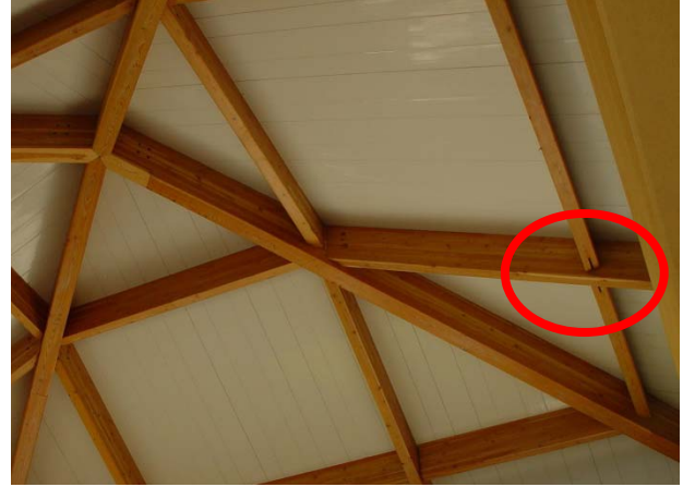
Figure 4: Steel knife plate slot extended to bottom of member. The slot in all other members is from the top only for better appearance
